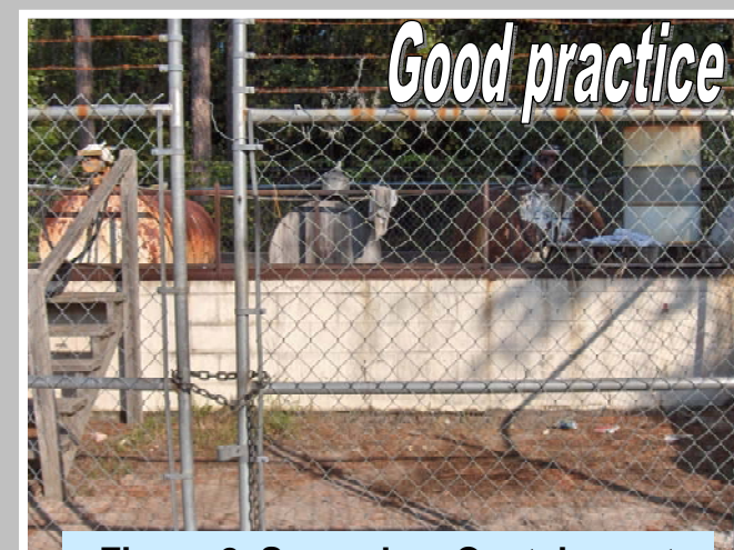
Figure 2. Secondary Containment
