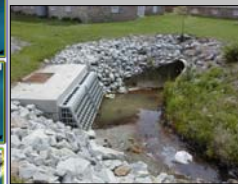
Figure 2. Yaupon Drive drainage basin on the South side of 25th Avenue South
